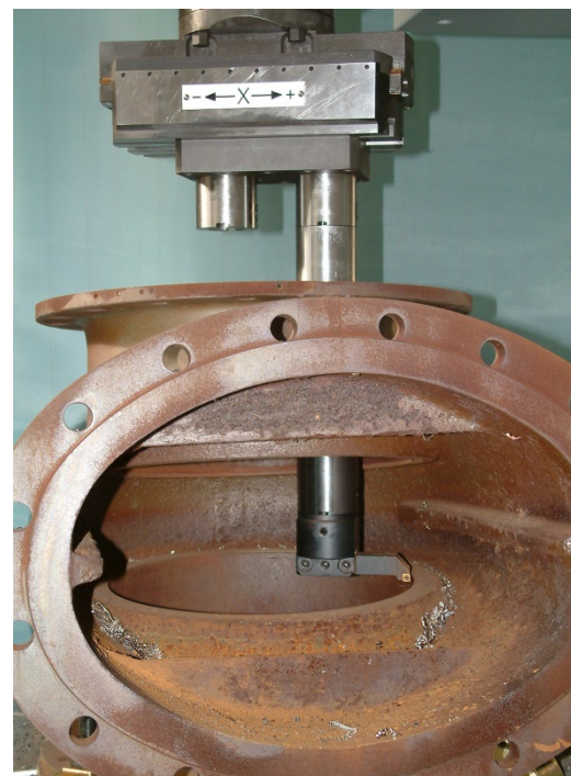
Face turning of sealing faces in valves and gate valves.
